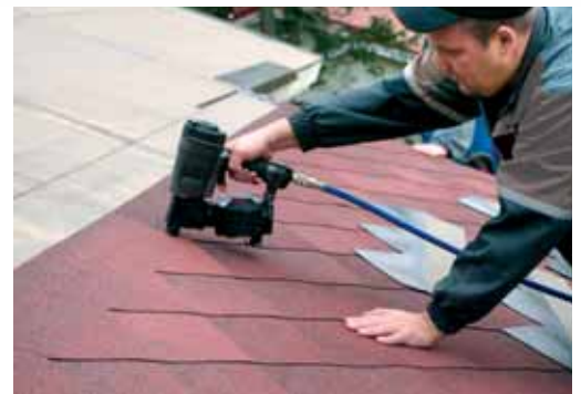
SuperFoxy shingles are installed.
